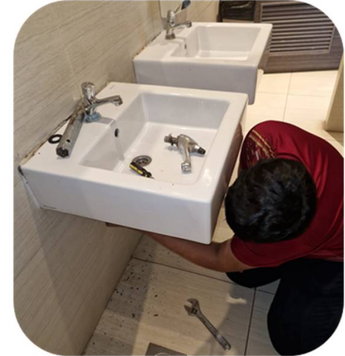
Replacing Water Faucet @ HomeTeam NS
