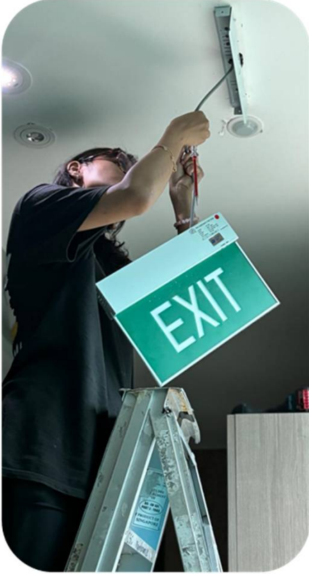
Installing Emergency Exit Light @ Civil Service Club
